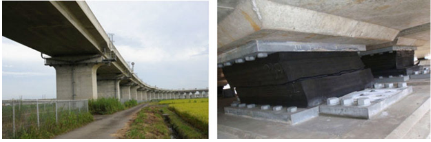
Fig. 5 Great East Japan Earthquake in 2011: bridge rubber bearings on the left and the horizontal crack is observed on the right [33]
