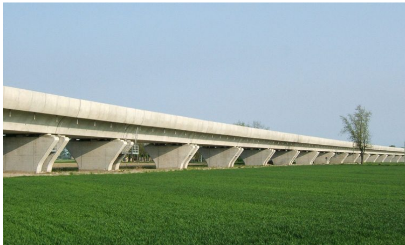
Figure 1. Railway viaduct in Piacenza, Italy (image taken from the website http://www.tensacciai.it , accessed on 31/01/2014). The structure is 5070 m long and consists of 150 prestressed concrete, simply supported spans. (Online version in colour.)
