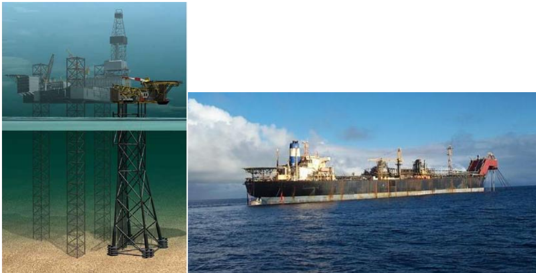
Figure 1 Fixed platform and Floating production system
