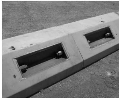
(d) Joint between two segments
