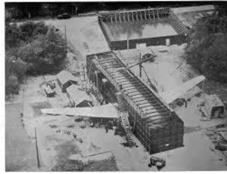
Fatigue test on the Comet G-ALYU fuselage (Farnborough, GB)
