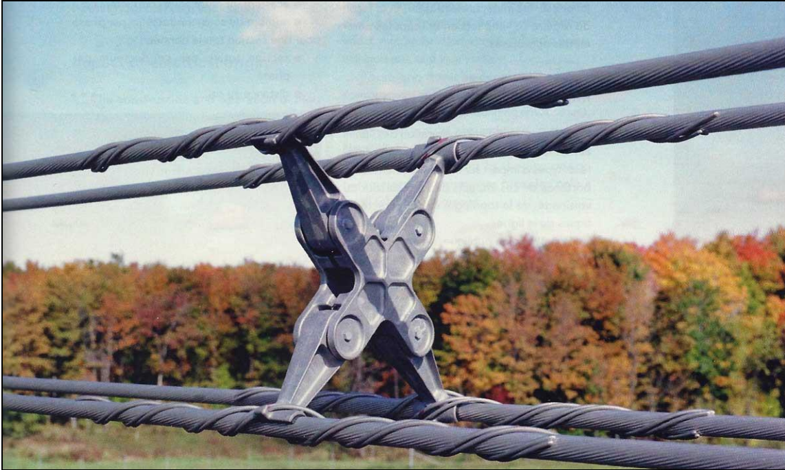
Fig. E-5. Hydro-Québec quad spacer-damper
