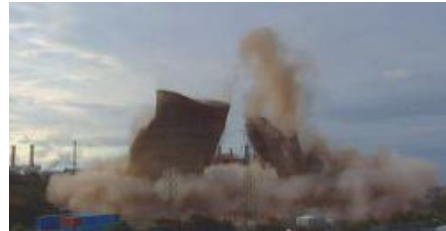
(b) Controlled collapse of each tower.
